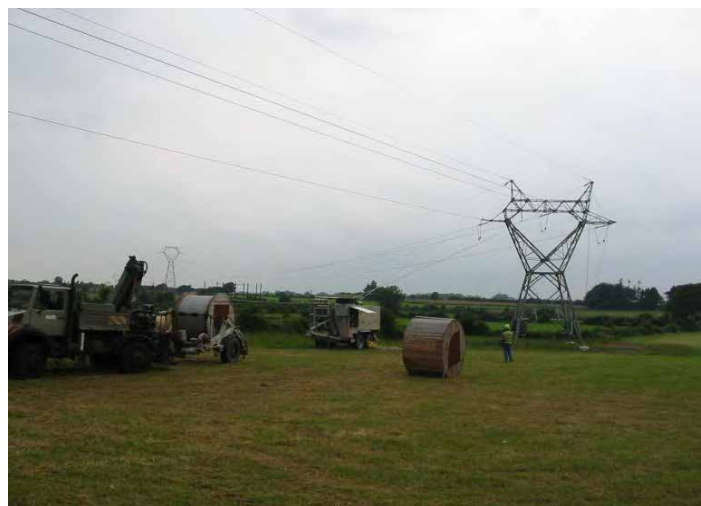
Figure 5.8 Typical Stringing Equipment
