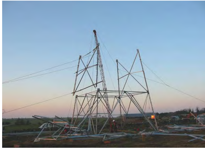
Figure 5.5 Derrick Pole at Tower Base
