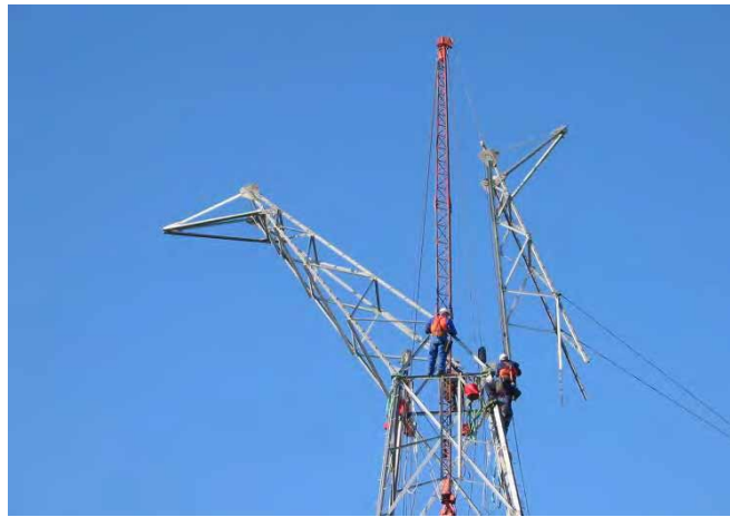
Figure 5.5 Derrick Pole at Tower Base
