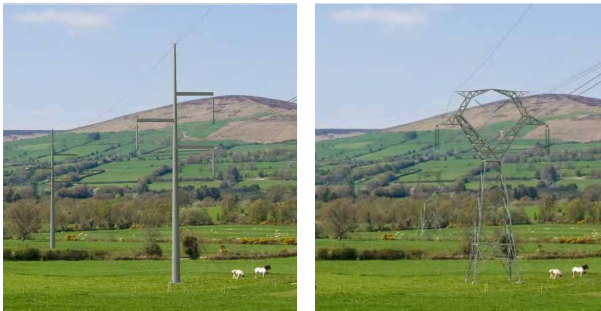
Figure 3.3 Atkins Monopole Design and Proposed IVI Lattice Tower
