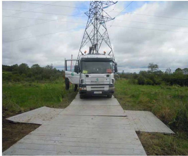
Figure 5.1 Temporary Aluminium Panel Tracks
